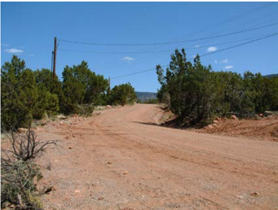
Dirt Residential Road (MRCOG)
